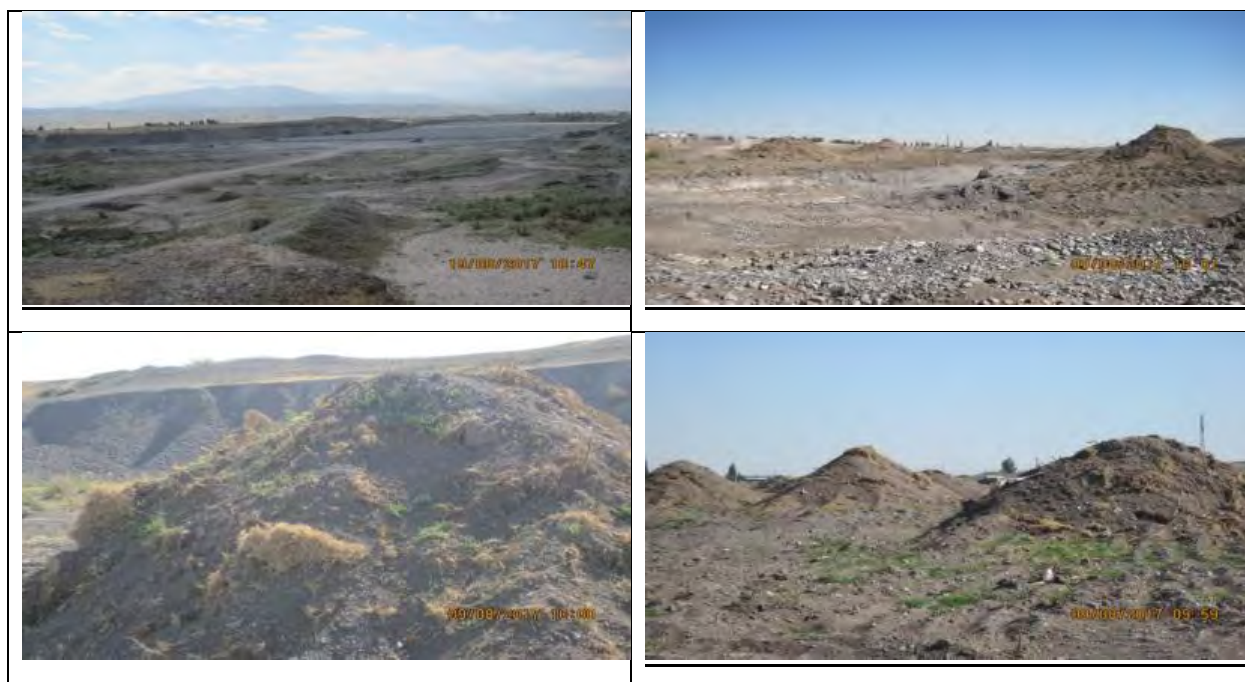
Figure 22 Ak-Suu1 borrow pit. Further, the removed soil layer was used for reclamation
