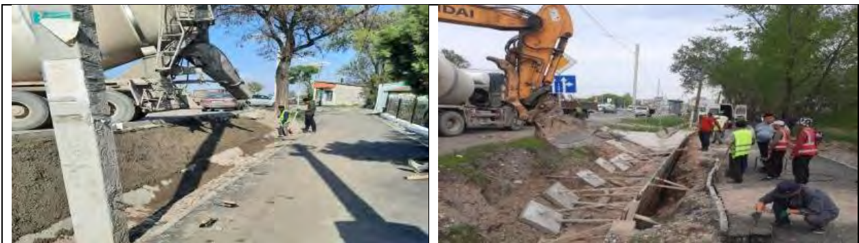
Figure 8 Strengthening of shoulders
