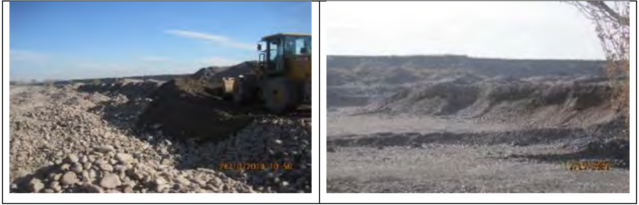
Figure 22 Development of Kara-Balta borrow pit
