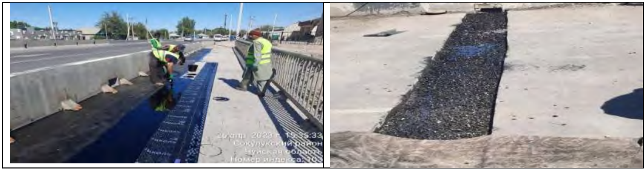
Figure 5 Construction work on the bridge over Sokuluk River
