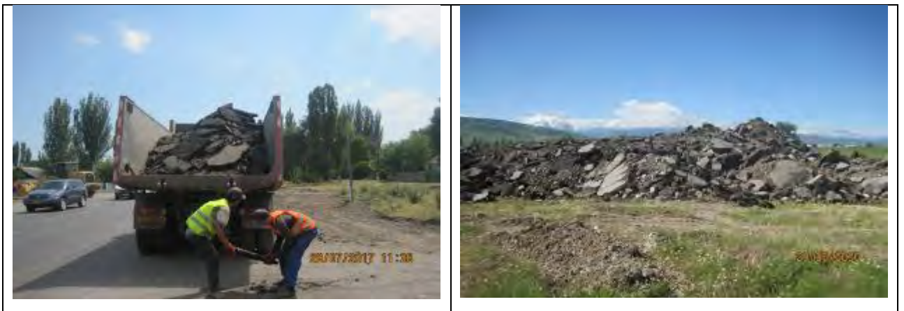
Figure 27 Old asphalt removed from the roadbed
