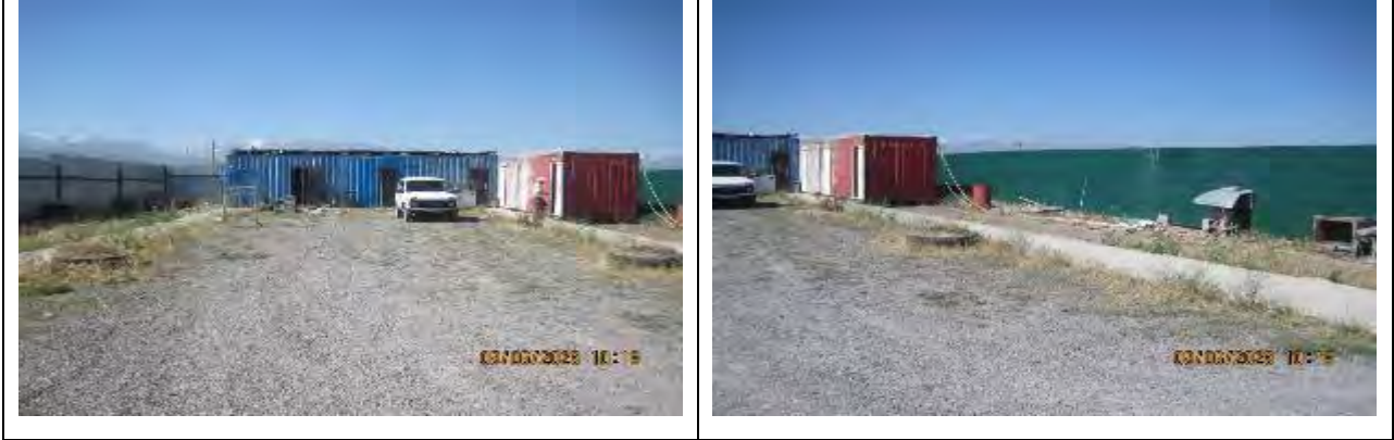
Figure 75 Dismantled camp for workers on the territory of the production site
