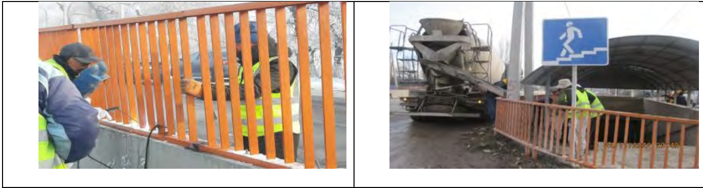
Figure 42 Installation of a metal grating near underpasses
