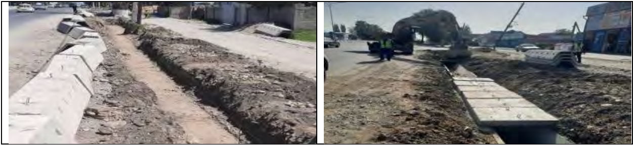
Figure 11 Installation of drainage ditches and OP-1 slabs above the ditches
