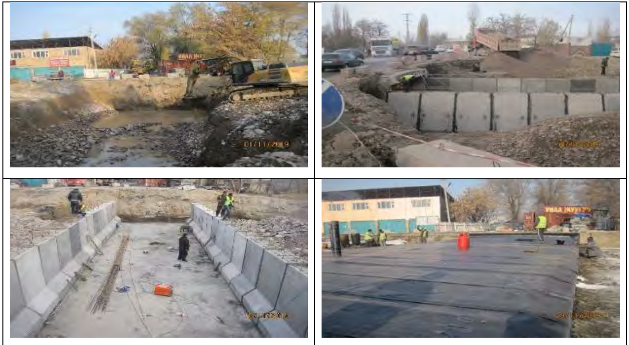
Figure 44 Construction of a bridge on the Jantai Canal
