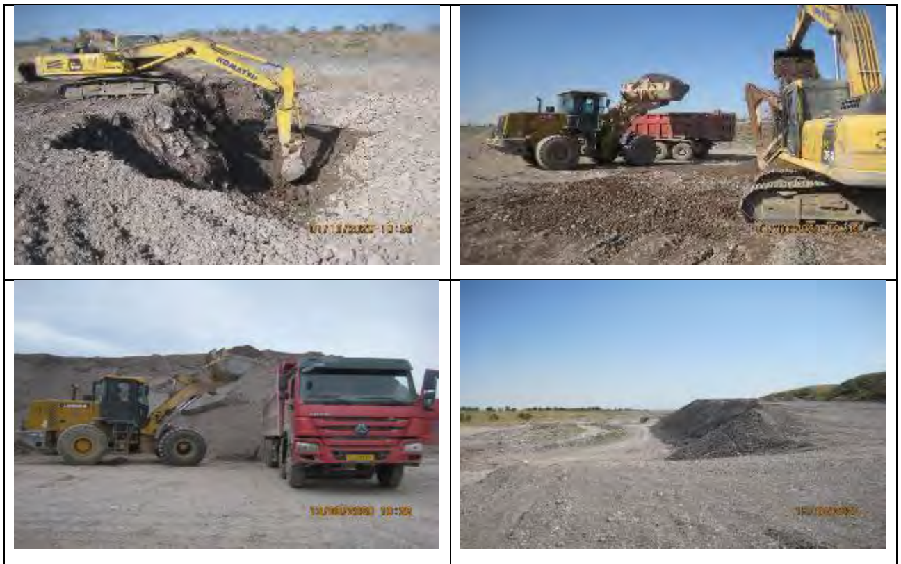
Figure 18 Development of the Ak-Suu 2 borrow pit on moistened material
