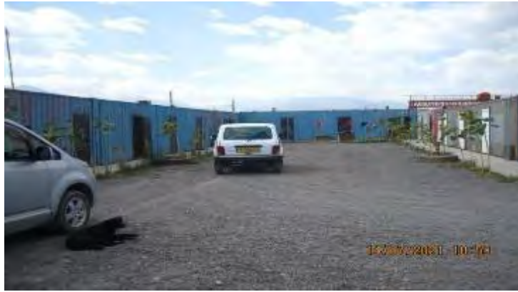
Figure 52 Workers' accommodation camp on the territory of the production site
