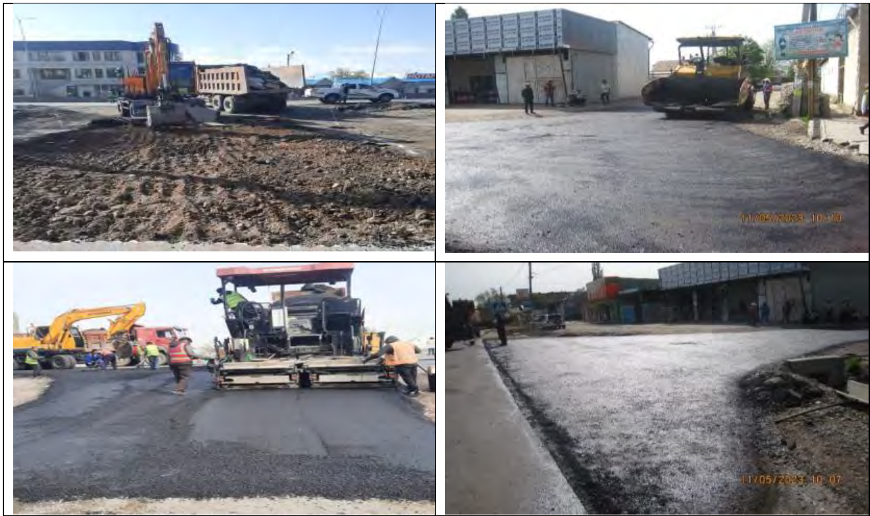
Figure 14 Construction of junctions to adjacent streets
