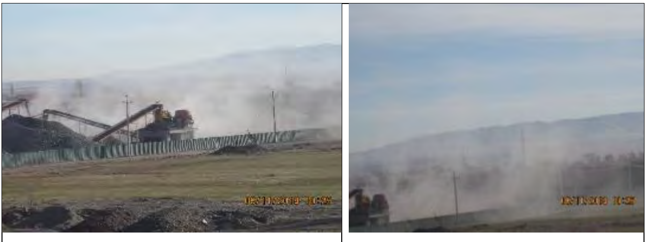
Figure 65 Dust in stone crushing plant
