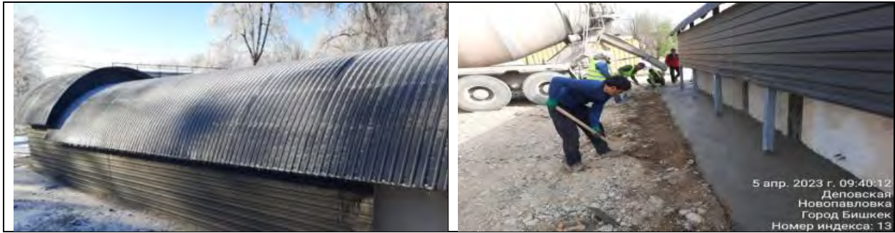
Figure 16 Work at the underpasses
