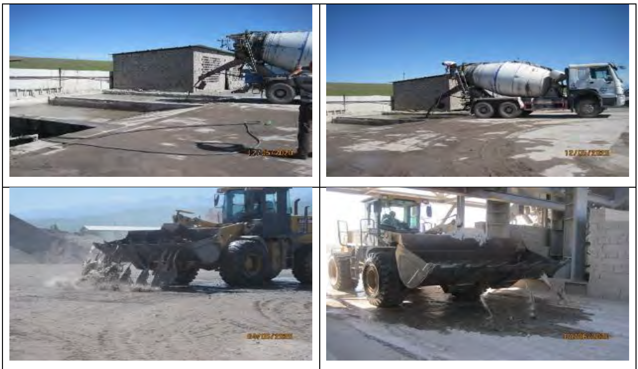
Figure 67 Washing of concrete mixers
