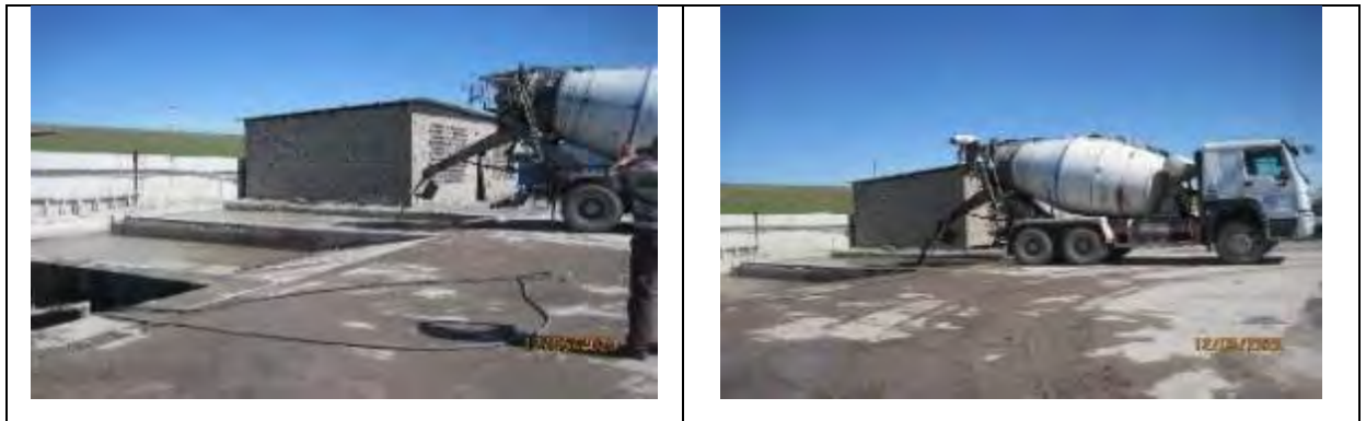
Figure 49 Washing of concrete mixer trucks
