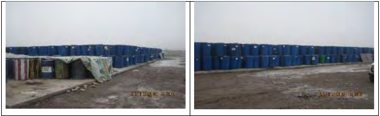
Figure 70 Bitumen in metal barrels stored on a prepared site
