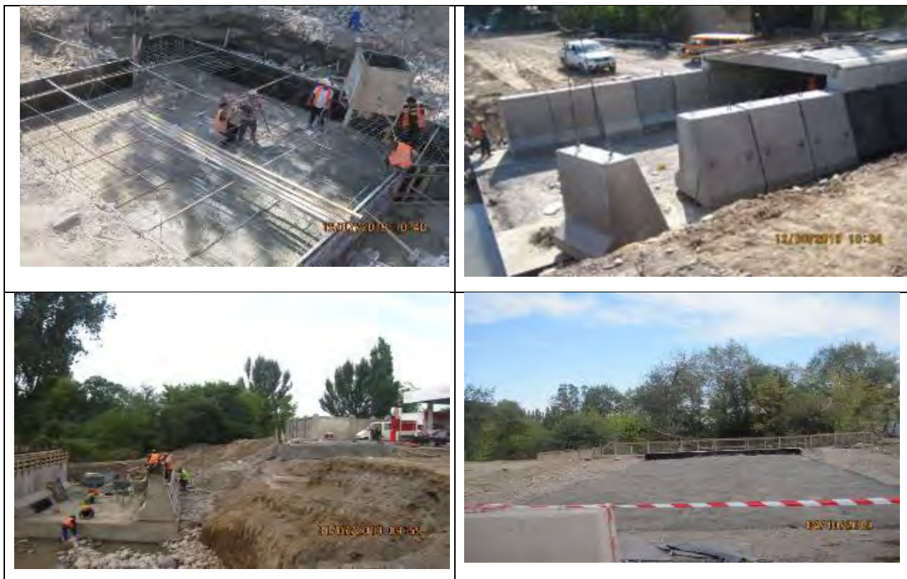
Figure 46 Construction of bridge on the Krepstnoy canal
