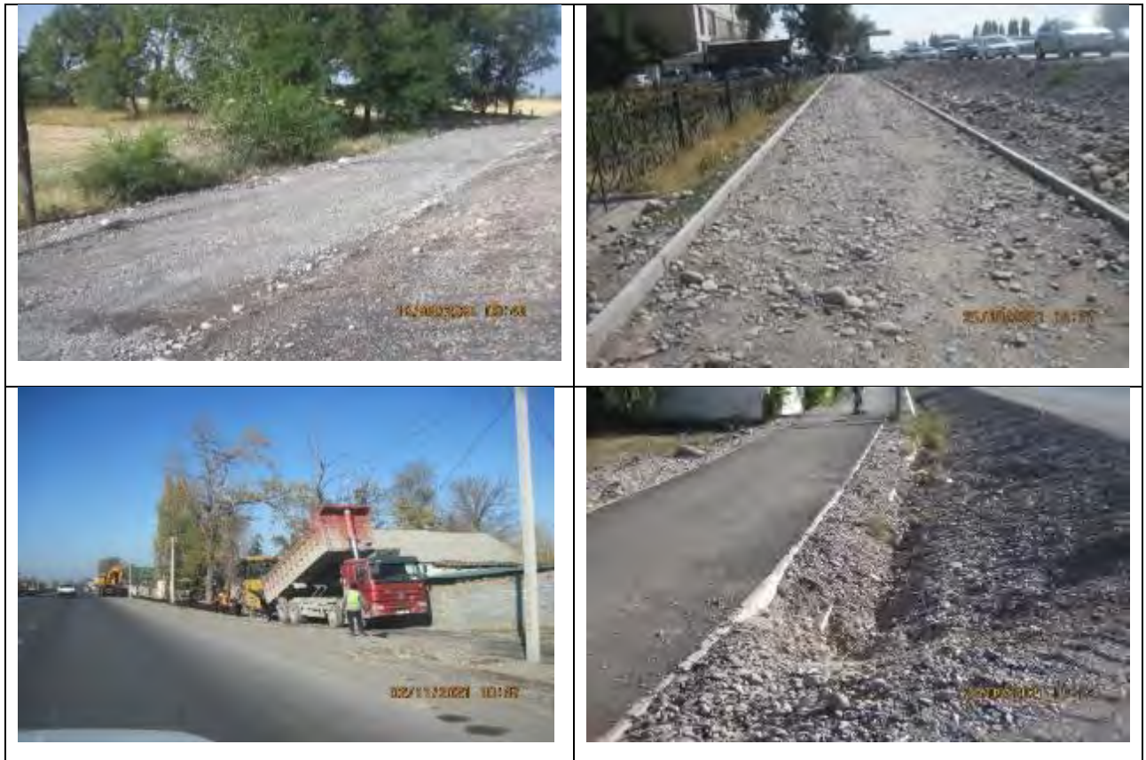
Figure 37 Construction of sidewalks
