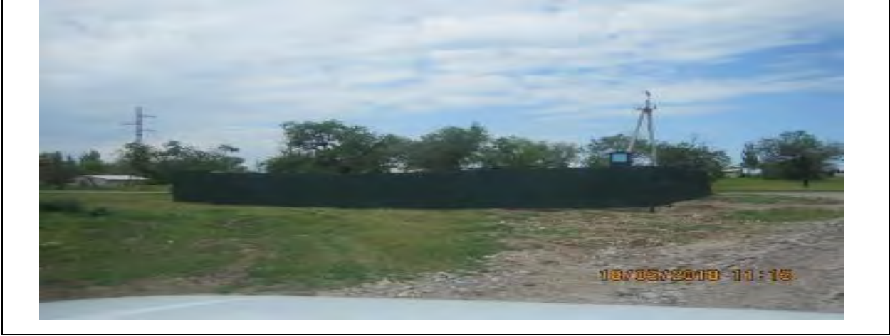
Figure 74 Restored well to supply the plant with water
