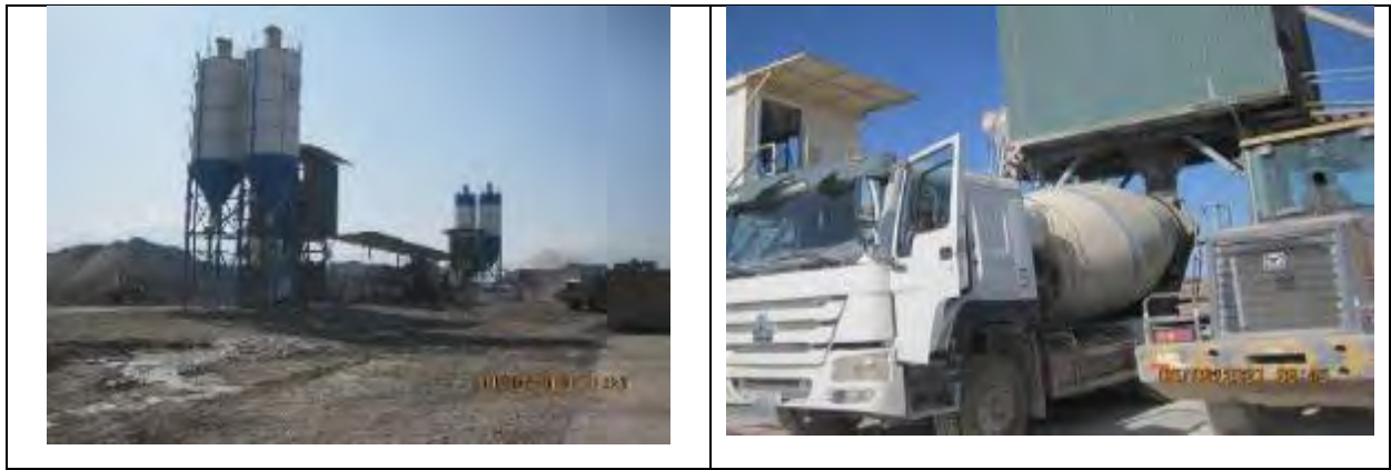
Figure 66 Filling the concrete mixing machine with concrete
