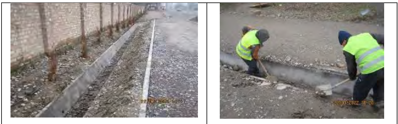
Figure 54 Cleaning of drainage ditches
