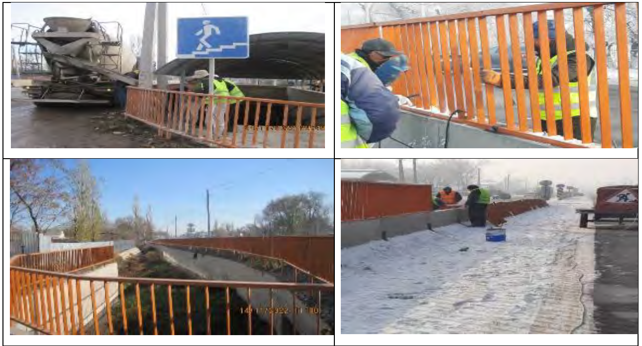
Figure 59 Installation of metal grating in road construction sites
