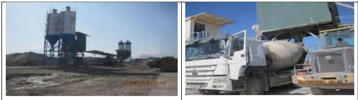
Figure 32 Filling the concrete mixing machine with concrete
