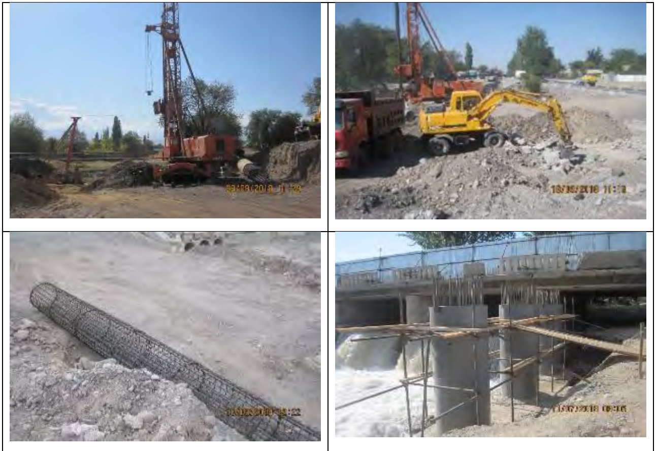
Figure 42 Construction of bridge across the Aksuu river
