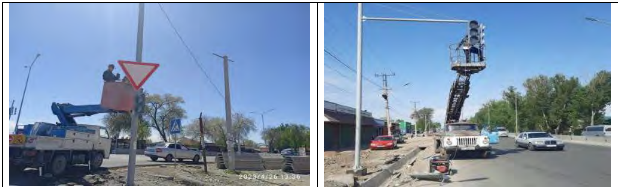
Figure 17 Installation of road signs and traffic lights
