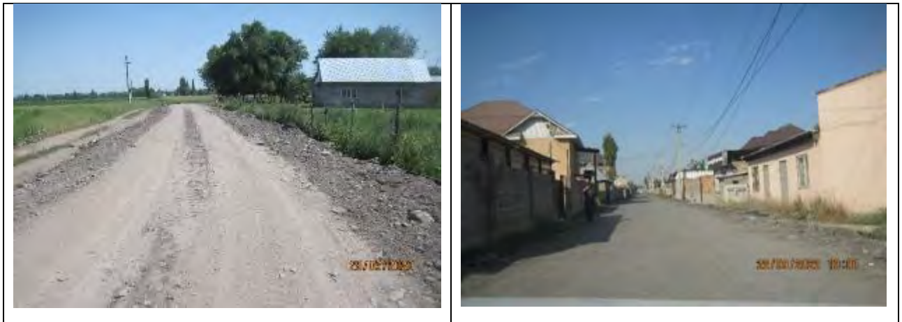
Figure 29 Streets backfilled with old asphalt
