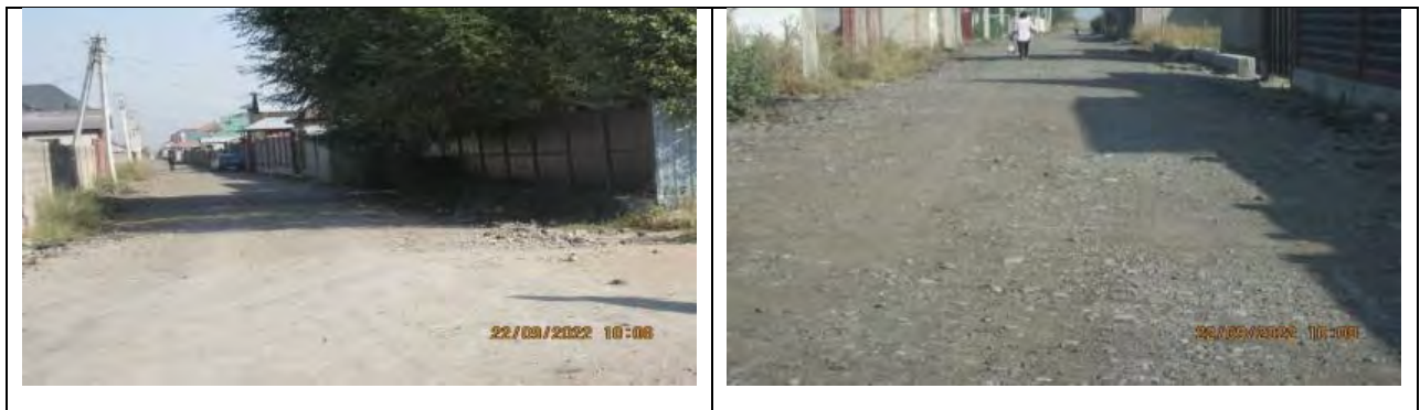
Figure 63 Streets paved with old asphalt at 7.4 km section
