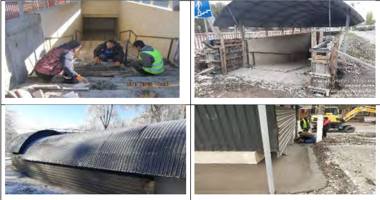
Figure 58 Construction works at the underpasses
