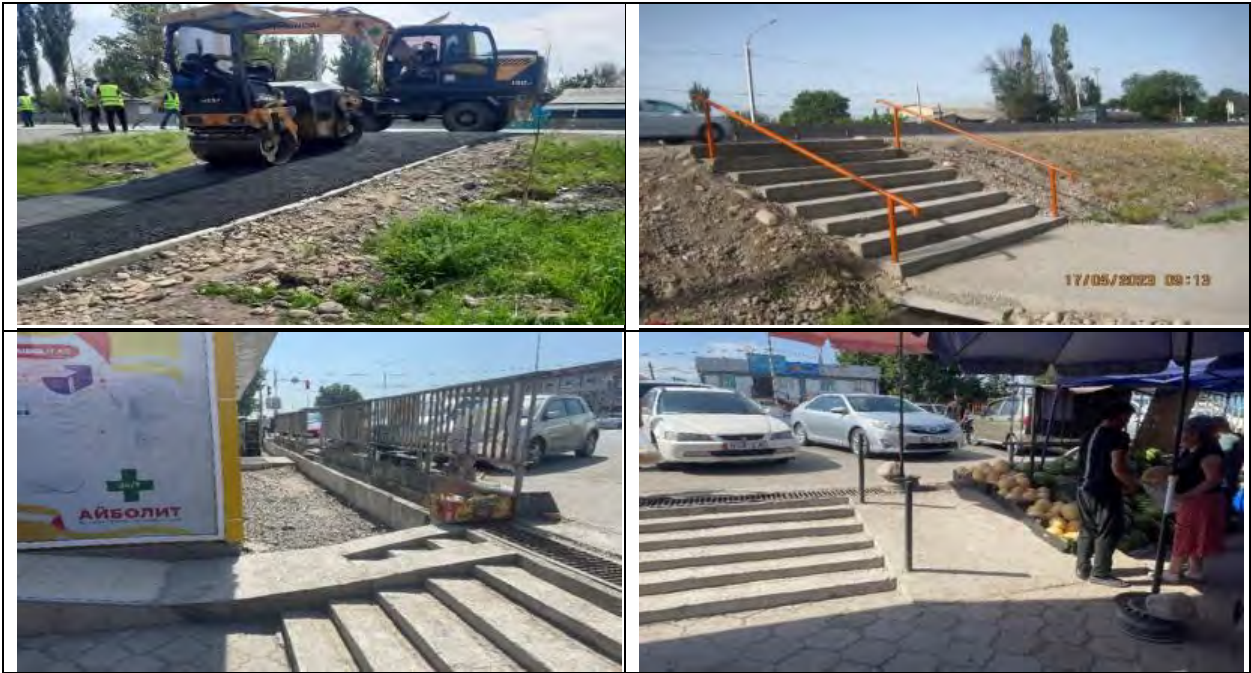
Figure 7 Construction of jointing walkways
