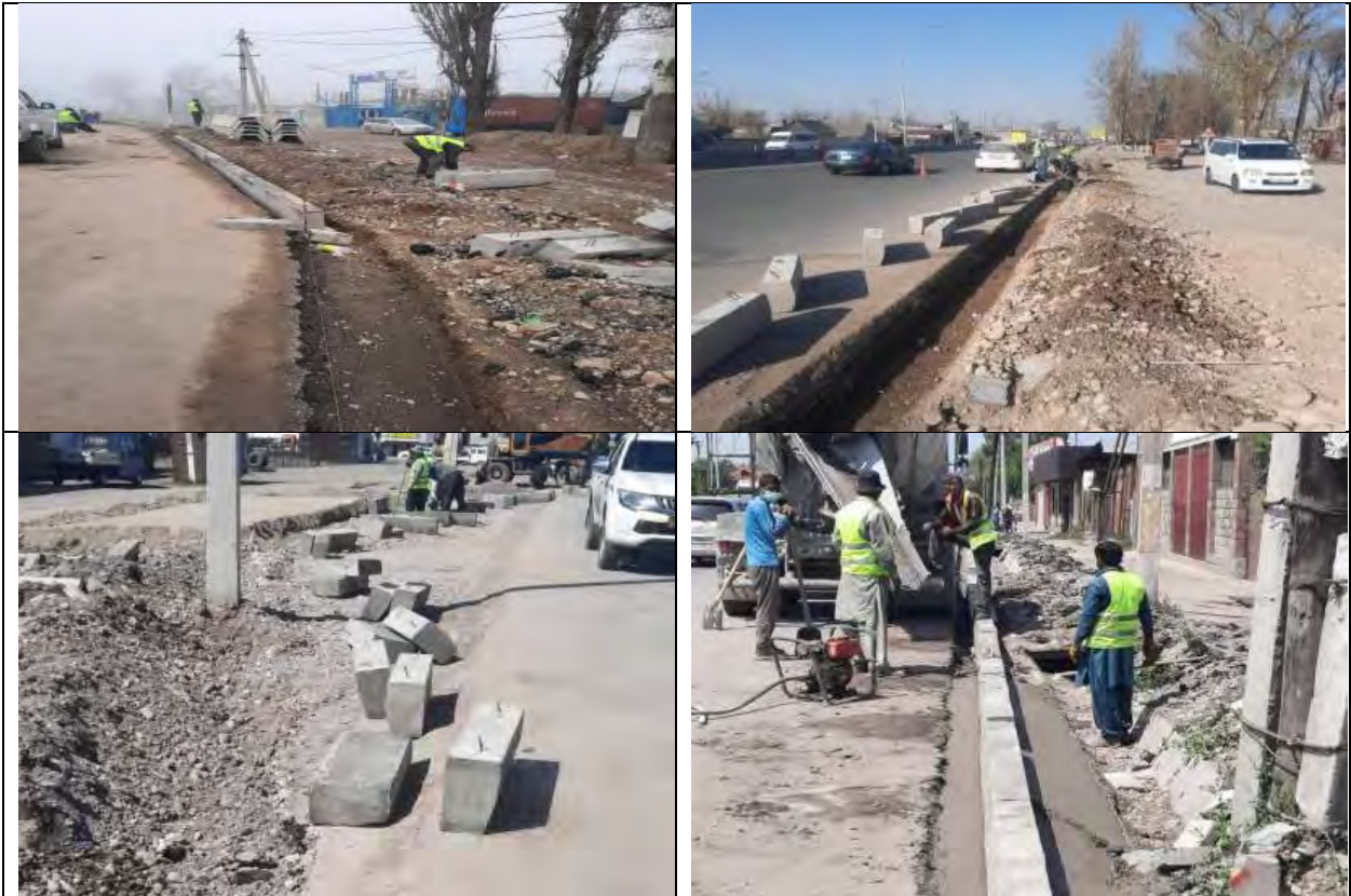
Figure 12 Installation of curb stones
