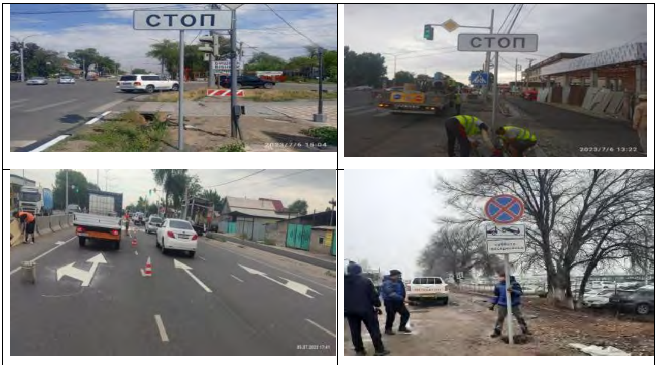
Figure 68 Installation of road signs and application of road marking
