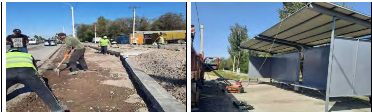
Figure 15 Construction of bus stops
