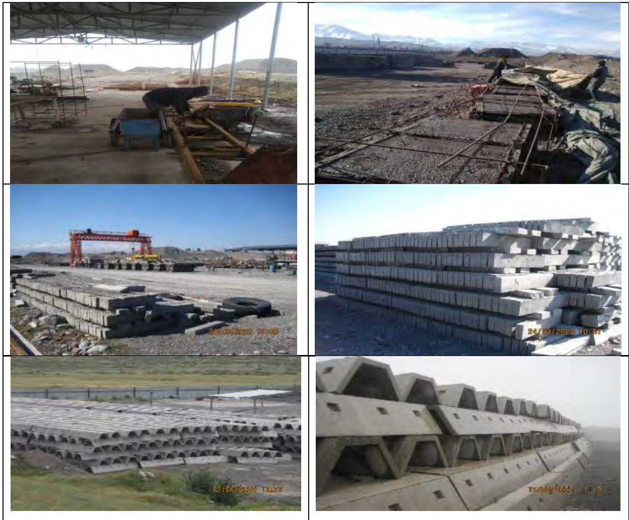
Figure 29 Manufacture of reinforced concrete structures at the plant
