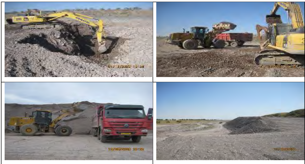
Figure 20 Development of the Ak-Suu 2 borrow pit on moistened material
