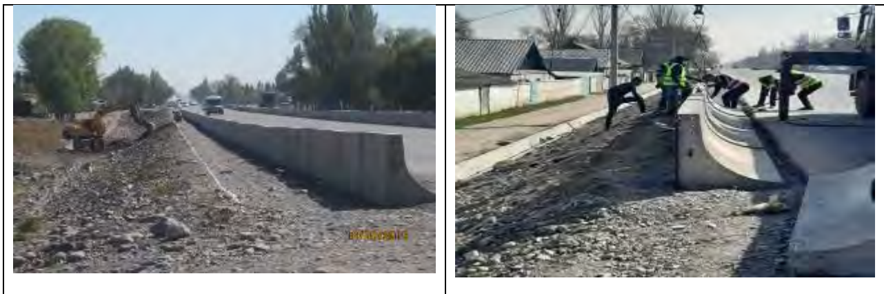
Figure 56 Installation of "Sapojok" type road curbs
