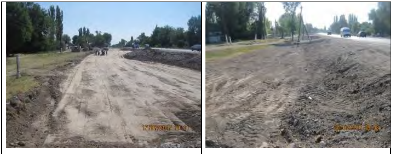
Figure 14 Road shoulders with removed topsoil
