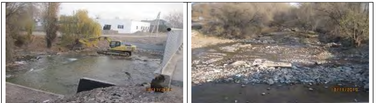
Figure 40 Cleaning the Sokuluk riverbed from construction waste
