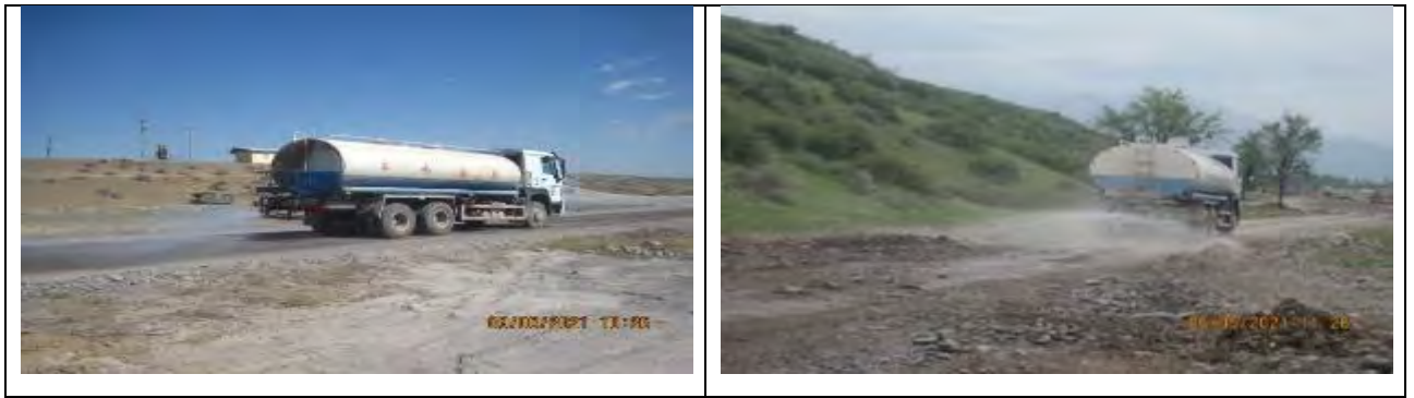
Figure 20 Water sprinkling on the access road to the Ak-Suu 2 borrow pit
