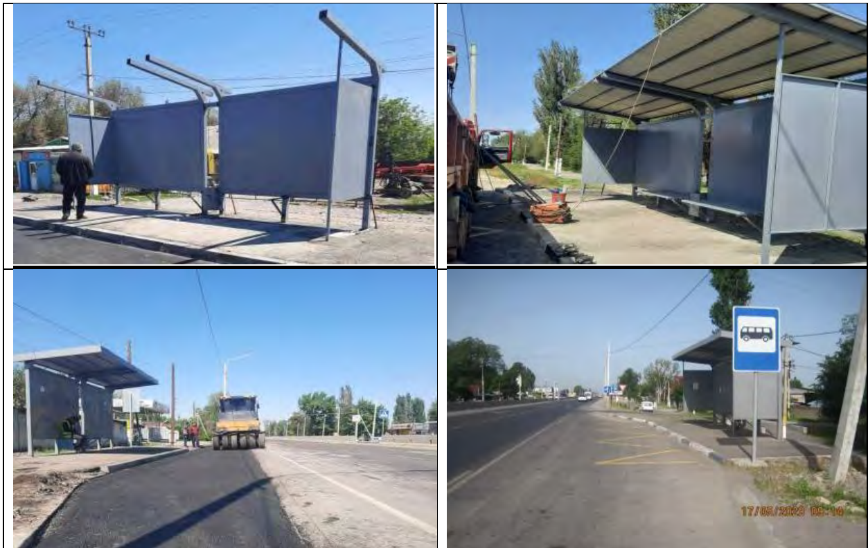
Figure 6 Construction of bus stop
