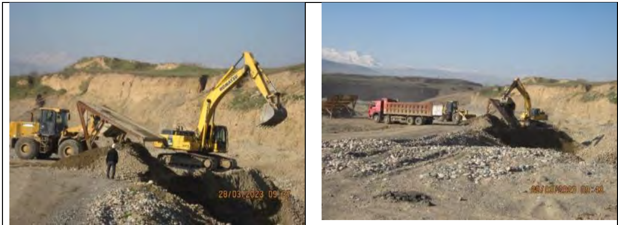
Figure 25 Development of Belek borrow pit
