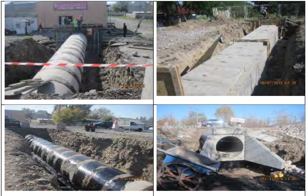
Figure 50 Construction of culvert pipes.
