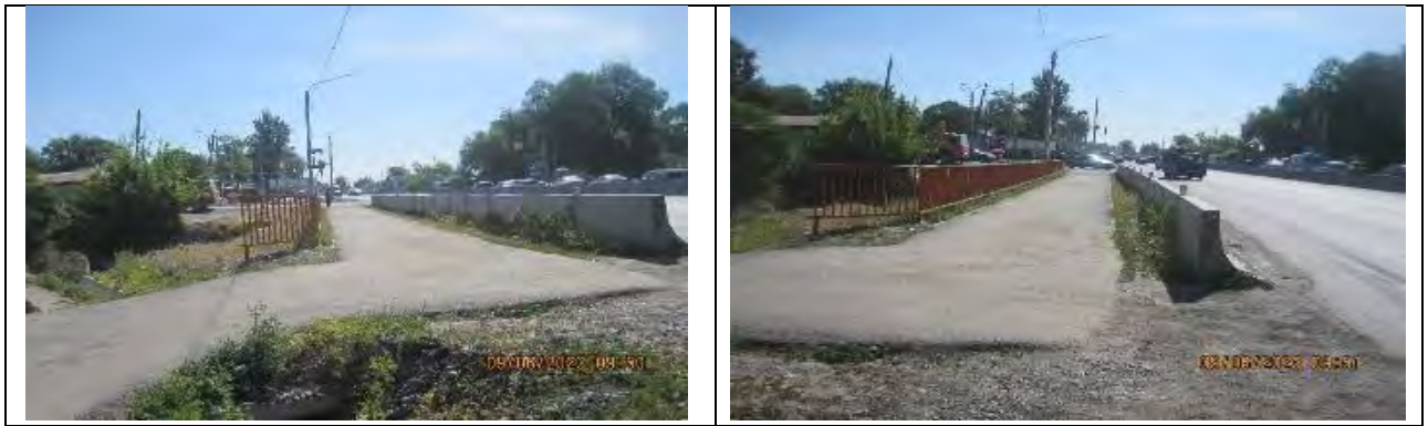
Figure 49 Pedestrian sidewalk on the new bridge at the Krepostnoy canal
