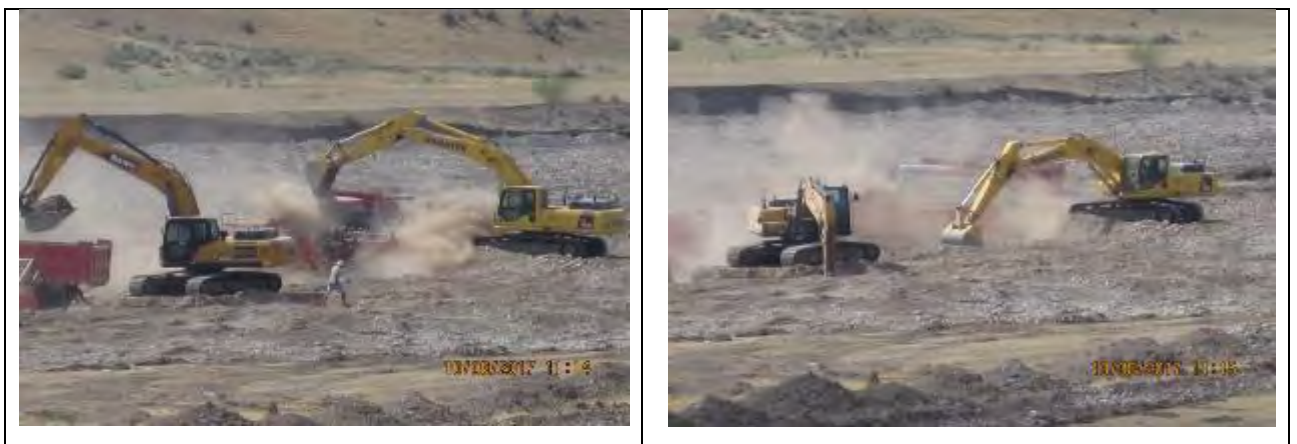
Figure 17 Dusting during work at the Ak-Suu 2 borrow pit. In the foreground, the removed soil layer
