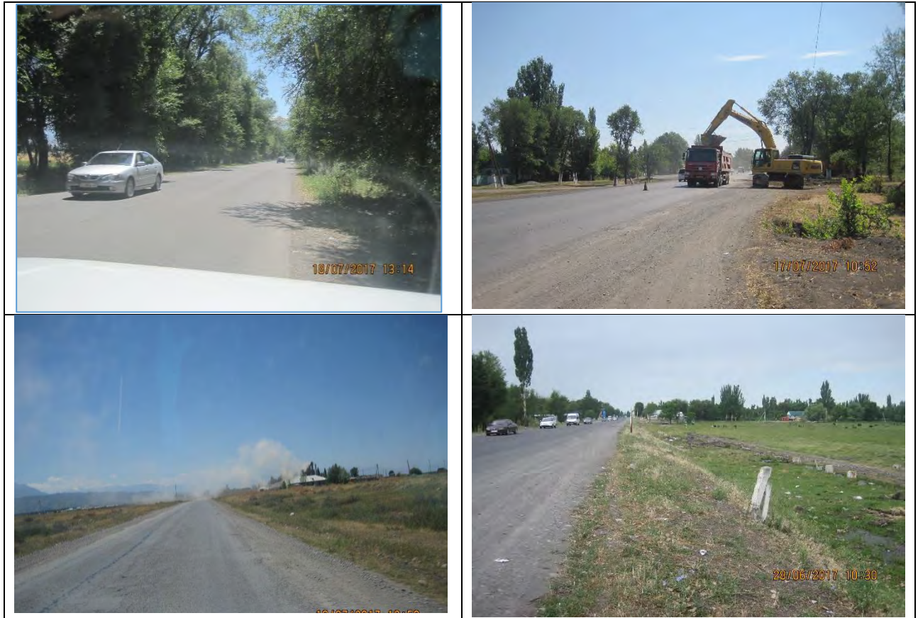
Figure 3 Bishkek Kara-Balta project road section, km 15.9 – km 61 before construction
