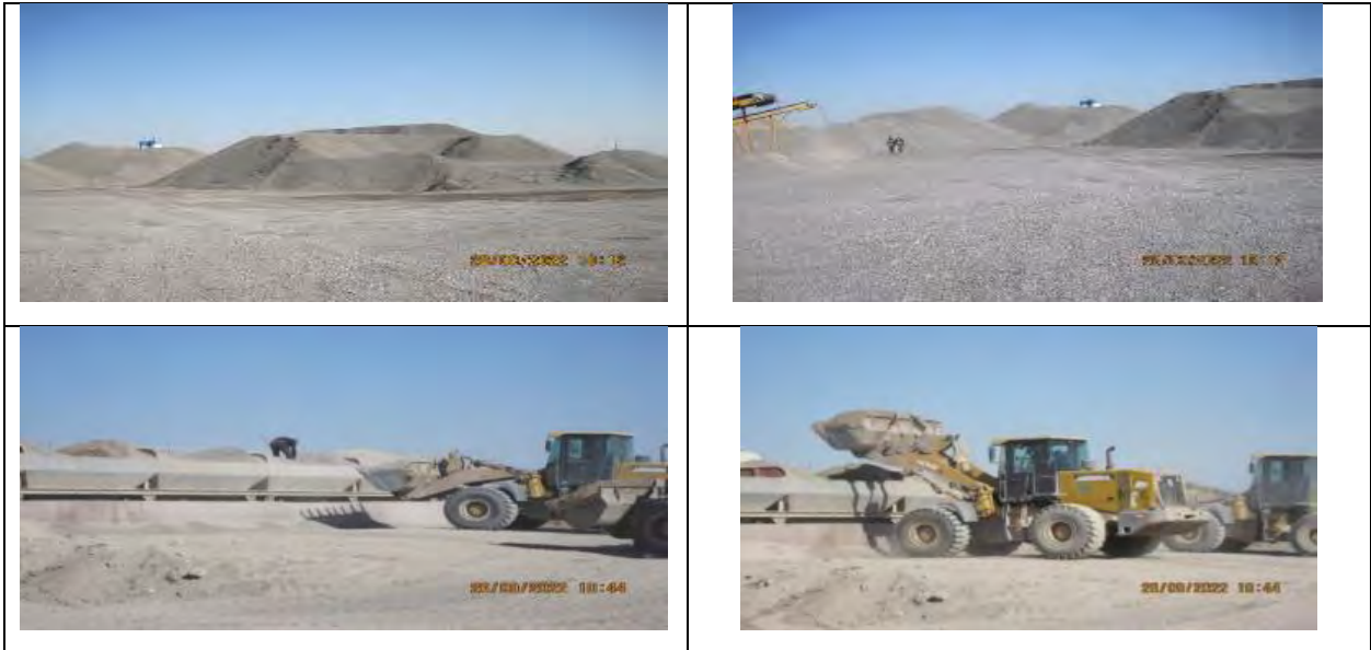
Figure 31 Preparation of gravel material for the production of concrete and asphalt
