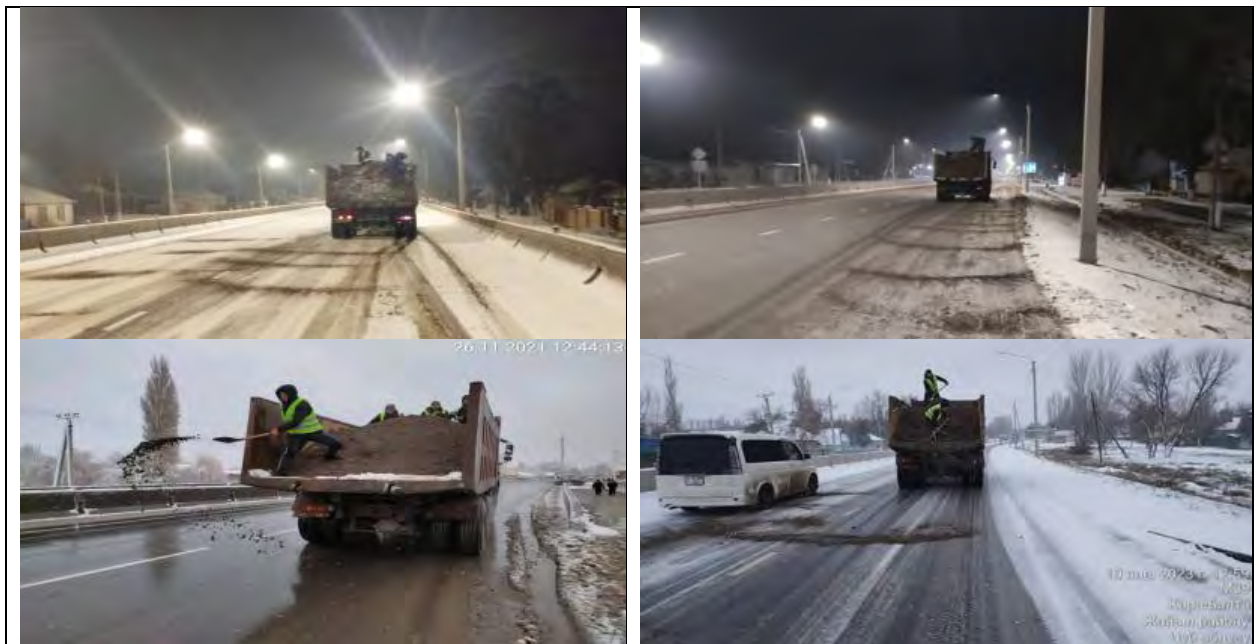
Figure 36 Sand sprinkling on the road. Control of ice
