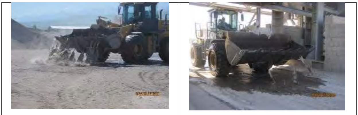
Figure 50 Watering of the production site with flushing water
