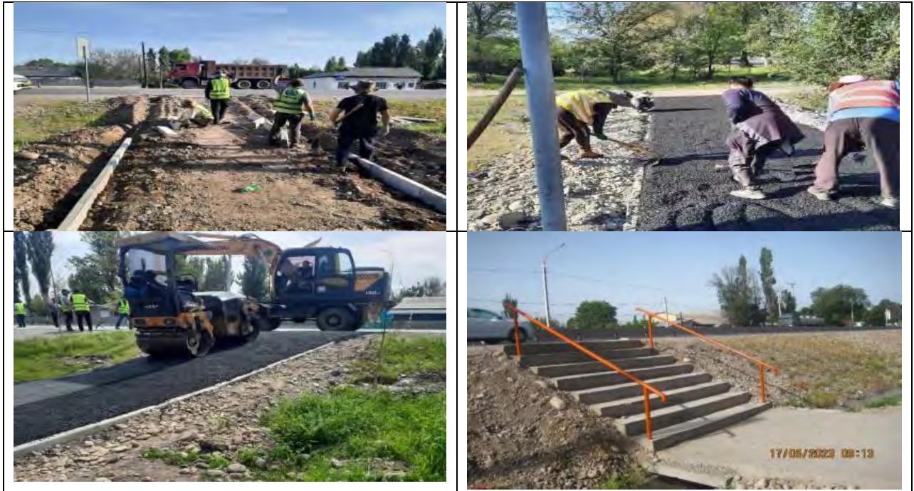
Figure 40 Construction of jointing walkways
