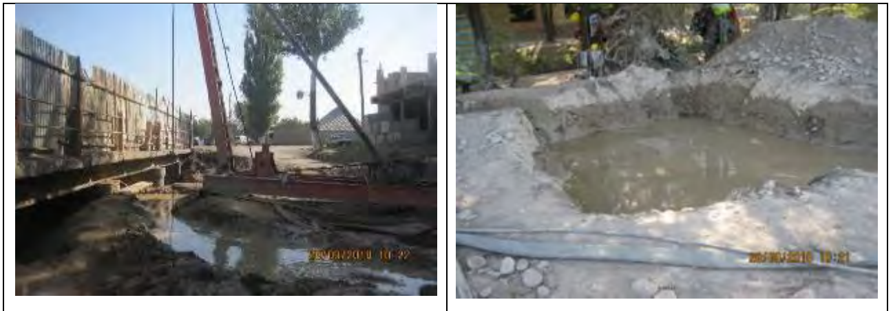
Figure 39 Construction of a bridge across the Sokuluk river. Bentonite pit
