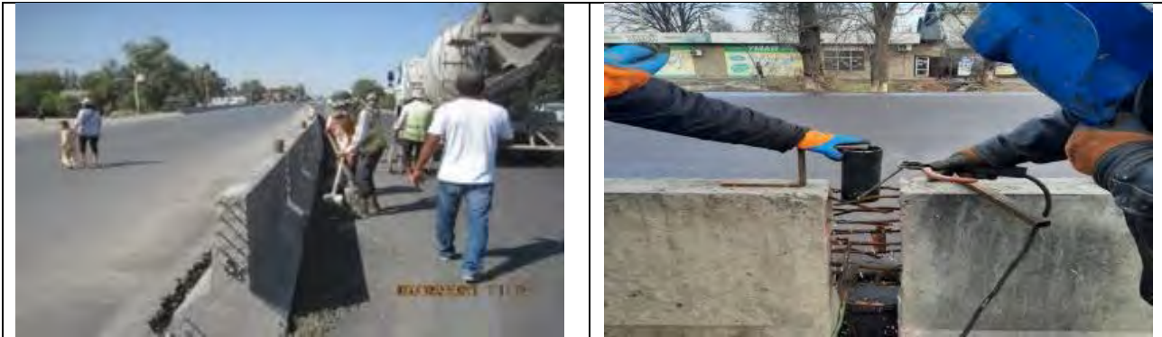
Figure 39 Works on concreting cuts on passages between parapets
