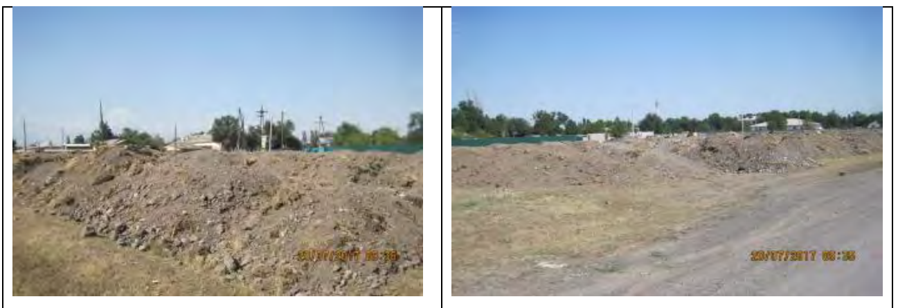
Figure 15 Dumps with removed and disposed soil
