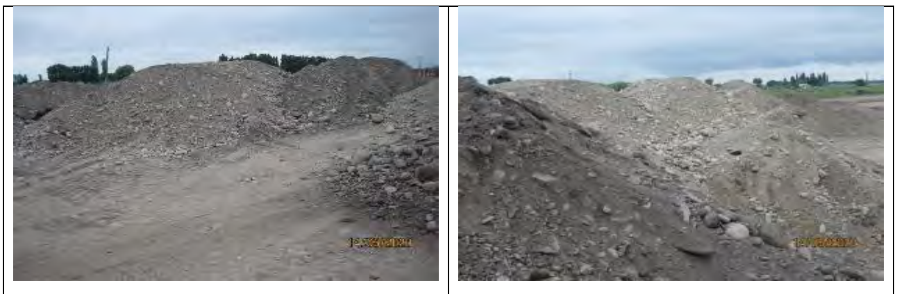
Figure 30 Storage of unsuitable soil for further use
