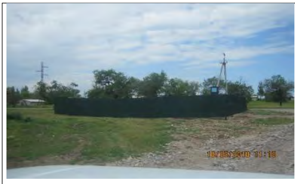
Figure 55 Restored well to supply the plant with water
