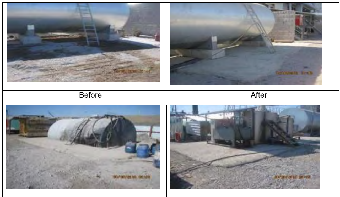
Figure 51 Impenetrable protective coating around chemical containers
