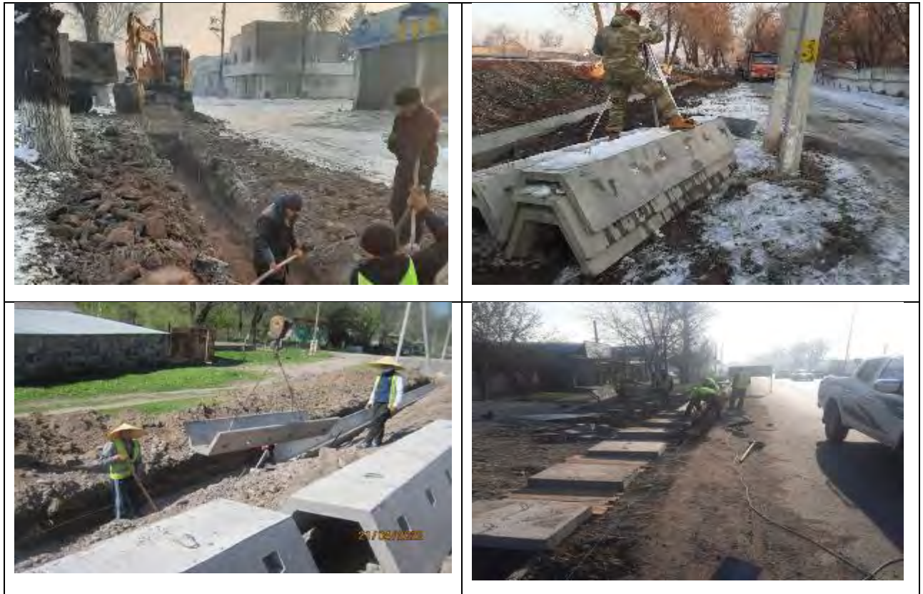
Figure 53 Construction of drainage ditches
