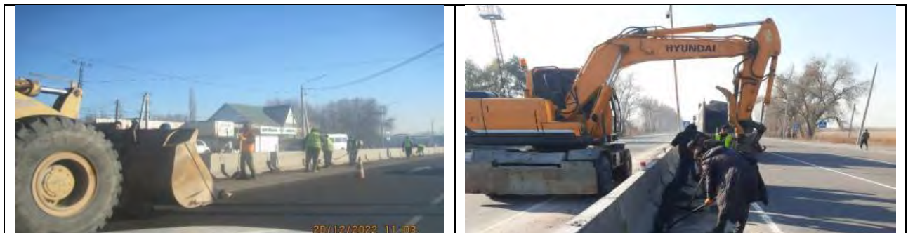
Figure 37 Cleaning parapets from soil waste and removal of waste from the road
