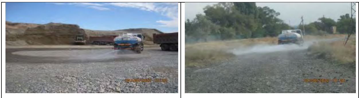
Figure 26 Dust suppression (water sprinkling). Road to the Belek borrow pit
