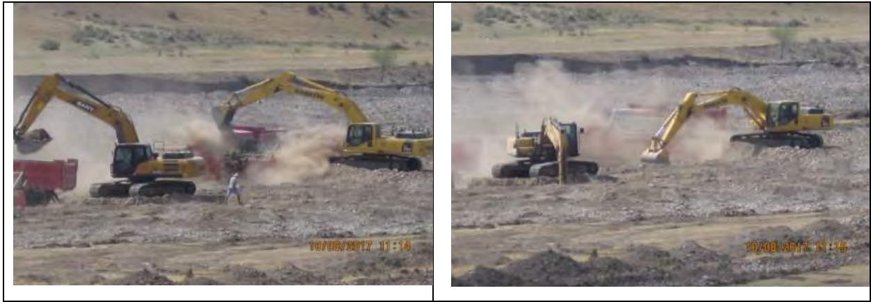
Figure 19 Dusting during work at the Aksuu 2 borrow pit. In the foreground, the removed soil layer.
