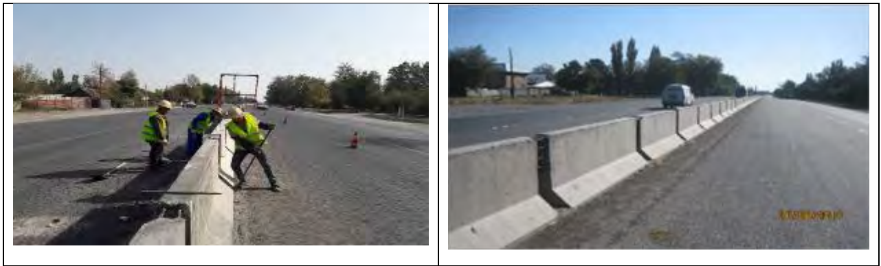
Figure 55 Installation of New Jersey type barriers.
