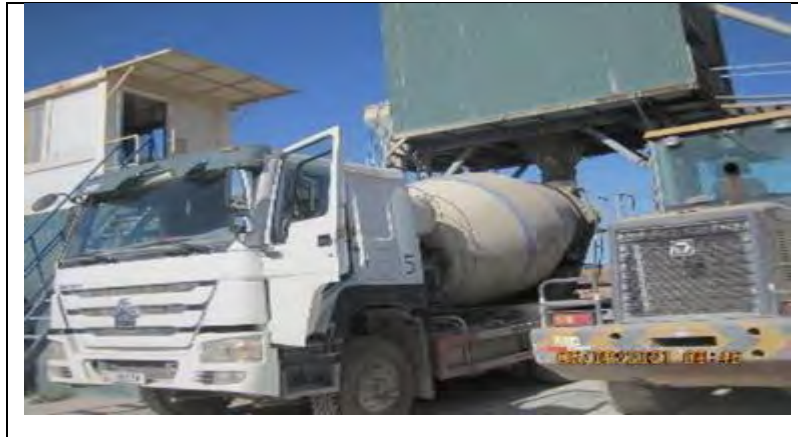
Figure 48 Refueling of concrete mixer trucks
