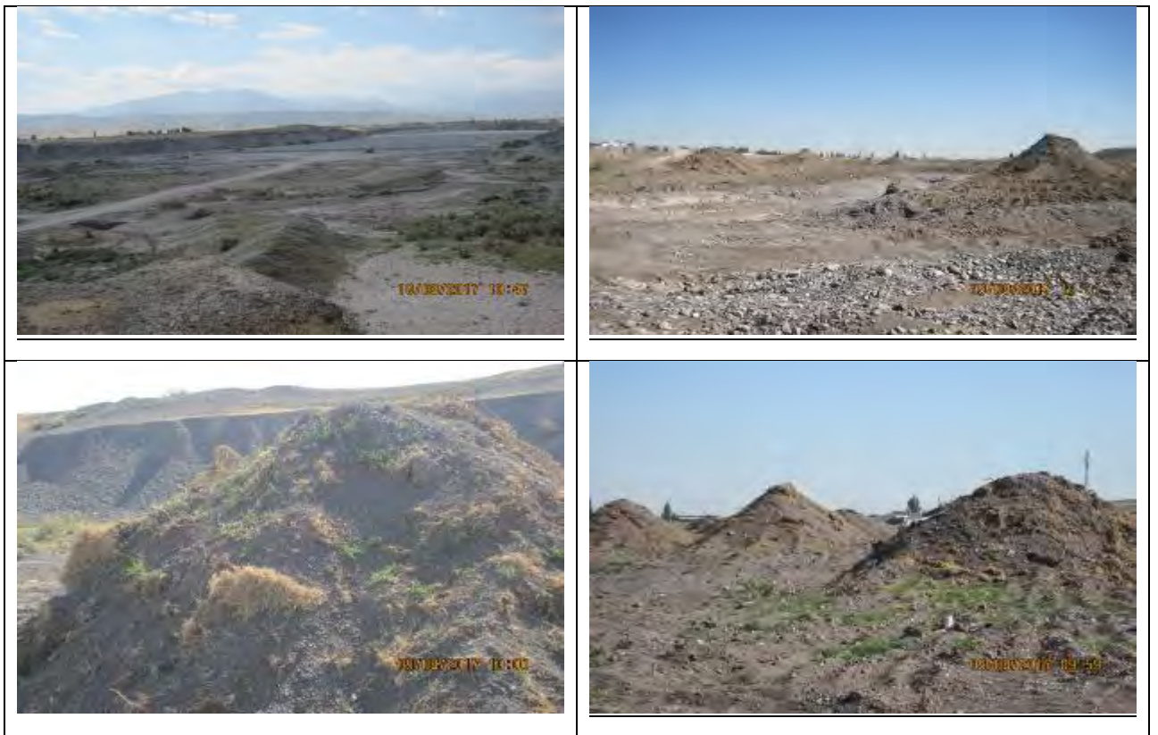
Figure 21 Ak-Suu 1 borrow pit. The removed soil layer was later used for reclamation.
