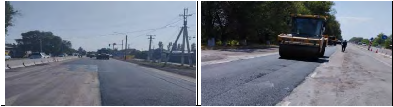
Figure 3 Milling and laying wearing course, removing ruts on the road
