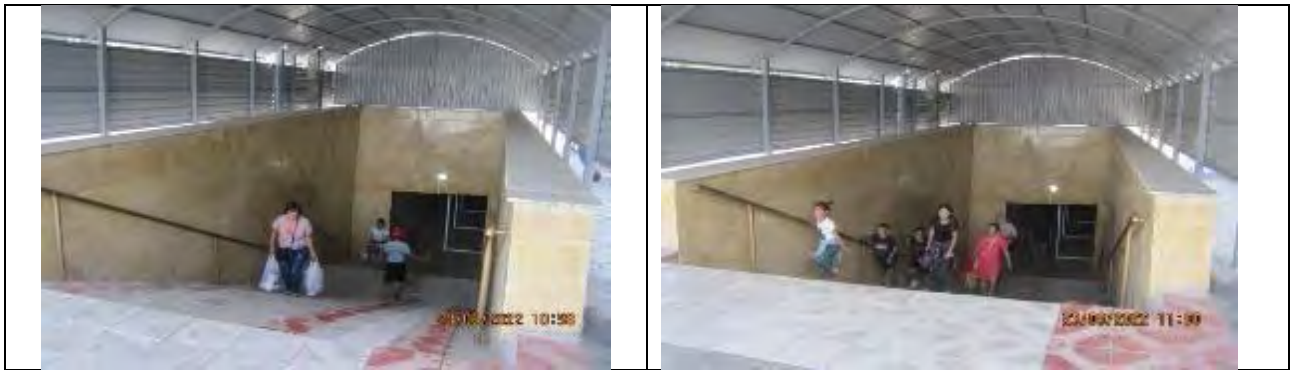
Figure 61 Underpass in the Sokuluk village
