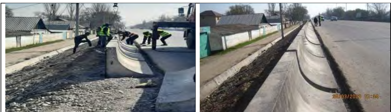
Figure 13 Intallation of curbs of Sapojok type
